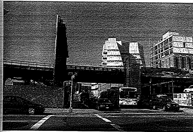
Photo 4 High Line railroad. In the background is the Frank Gehry-designed IAC headquarters (opened 2007), which was built under the pre-2005, manufacturing zoning. The new zoning is unleashing a wave of condominiums. Photo by Elisabeth Tiso.
